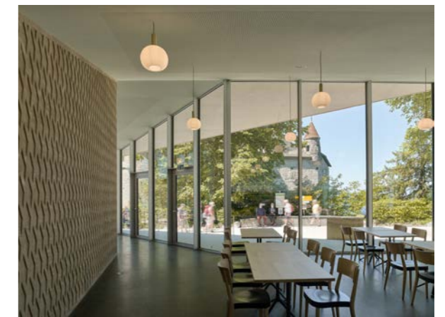
Jardin Anglais Cafe Pavilion. Glazing installed at varied angles reveals different views of surrounding garden
