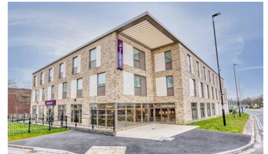
Premier Inn Peterborough City Centre
