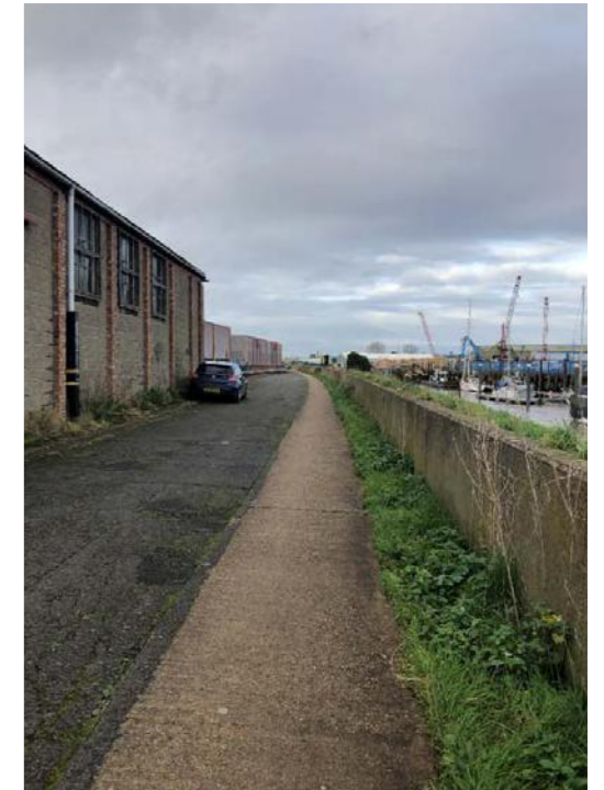
Warehouses/flood defences on West Parade
