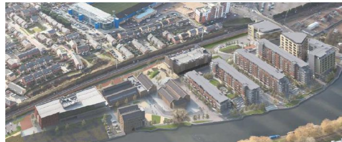
Precedent: Fletton Quays, Peterborough - NORR Consultants
