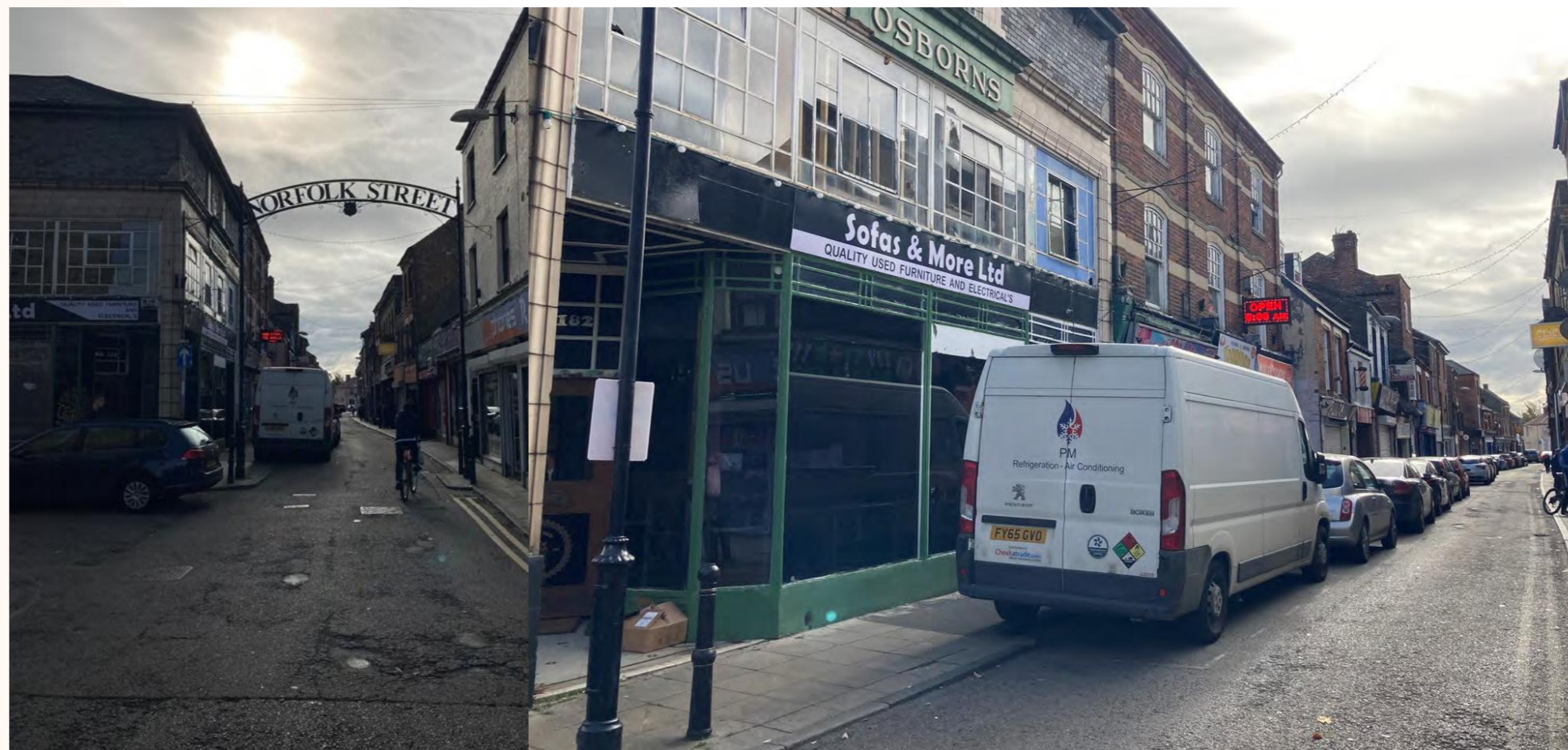
Views of the entrance to Norfolk Street and the existing public realm/street frontages
