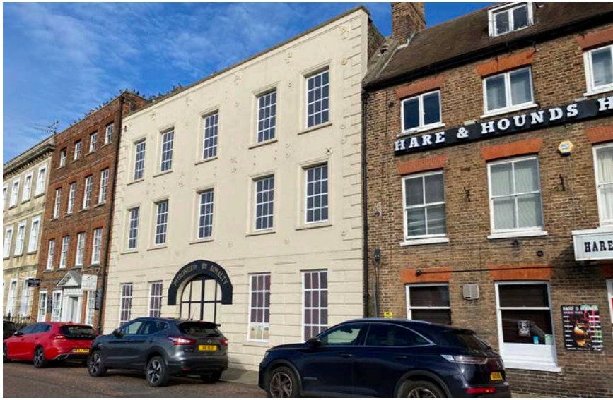
Phoenix Hotel facade - all that remains following a fire in 2010
