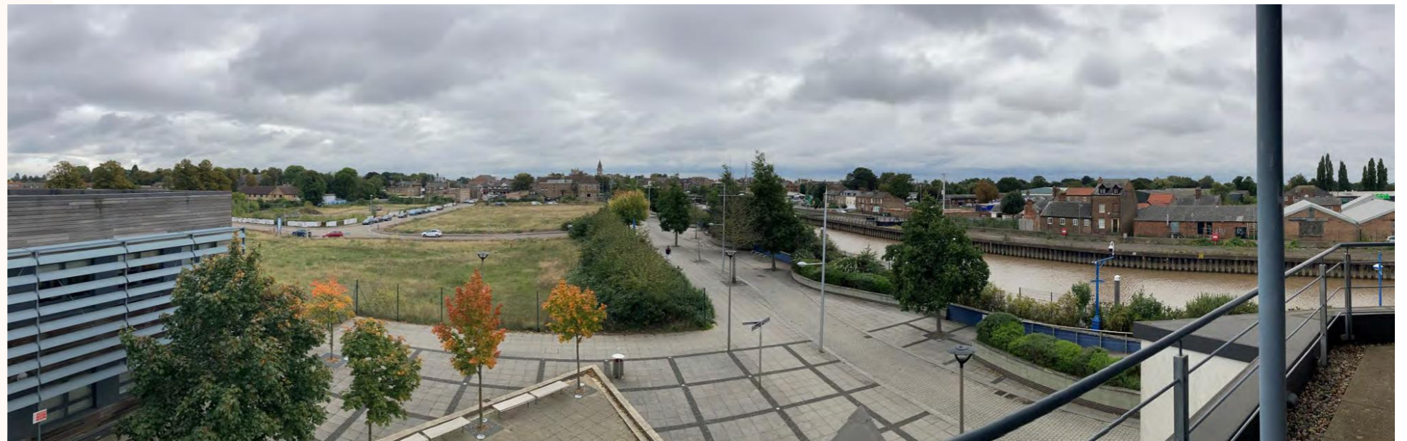
View from the Boathouse business centre overlooking Nene Parade and the development plots
