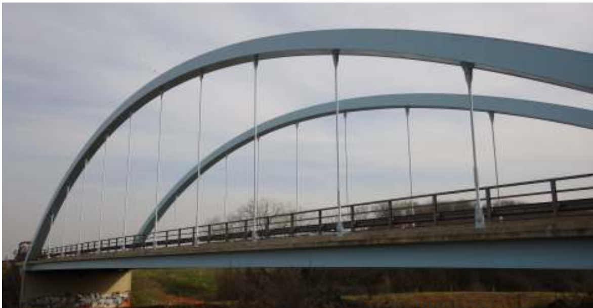
Figure 4.2 – Car Dyke Bridge, a steel tied arch bridge near Peterborough
