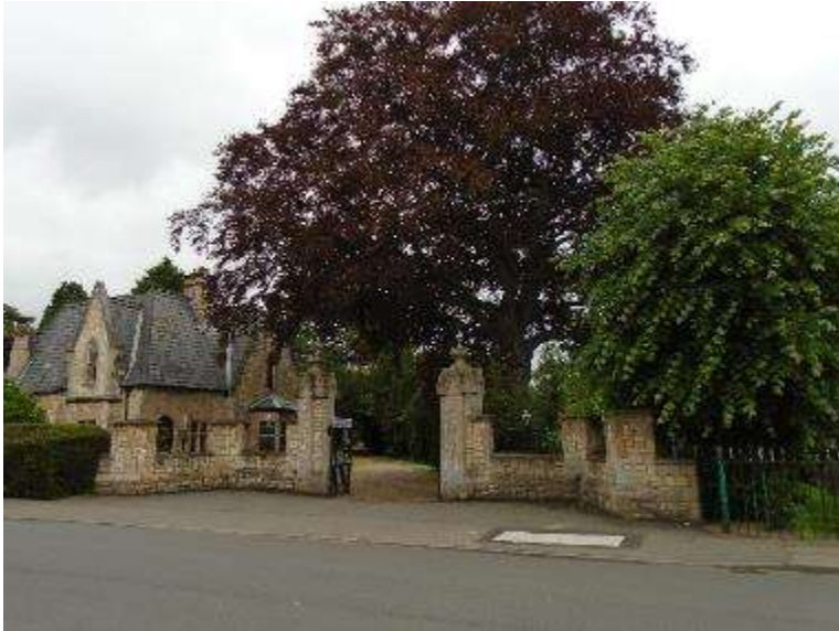
Looking east at the main entrance
