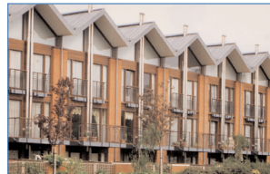
Fig 3.2: Residential may predominate, but it must be supported by a mix of other uses
